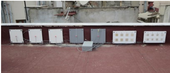
Figure 15: General view of the parapet wall with the samples installed at the case study building in Istanbul.
