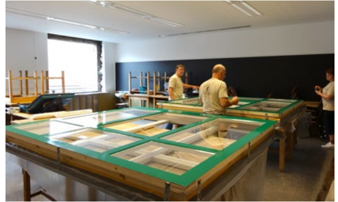
Figure 18: Installation in the case study building in Budapest
