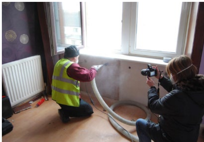
Figure 10: Installation of aerogel fibre insulation into test panels
