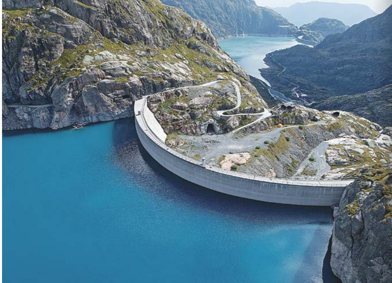
■ Reservoirs of the Nant de Drance pumped-storage power station. With an output of 900 MW, it will generate around 2.5 billion kWh of electricity per year when it commences operation at the end of 2018. © Michel Martinez, 2012
