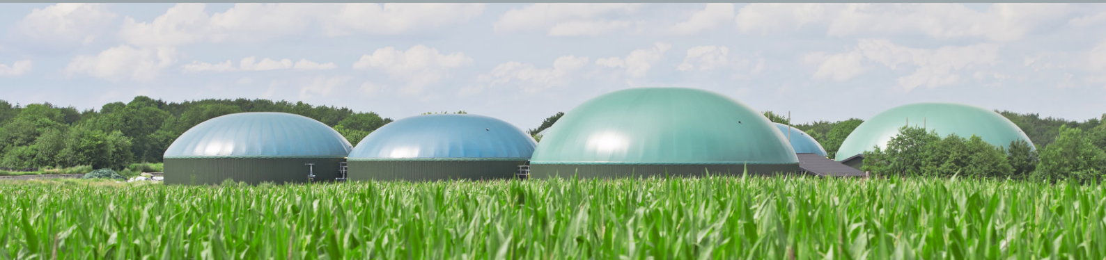
Modern biomass plant in Europe.
